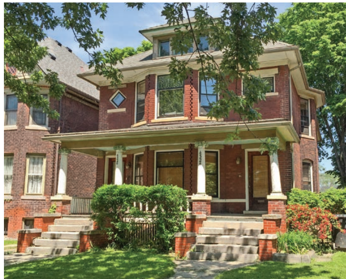
▲ A duplex (such as this one in Detroit, Michigan) can be so similar in form to a single-family house that sometimes the only clue is the presence of two entrances.
