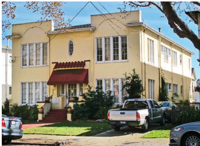
▲ Up until the 1940s, small, multiunit buildings (such as the Alameda, California, fourplex pictured here) were commonly built on standard lots within neighborhoods to provide housing for moderate-income individuals and families.
